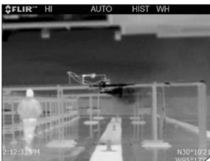
Ammonia (NH 3 ) gas escaping from pipes
